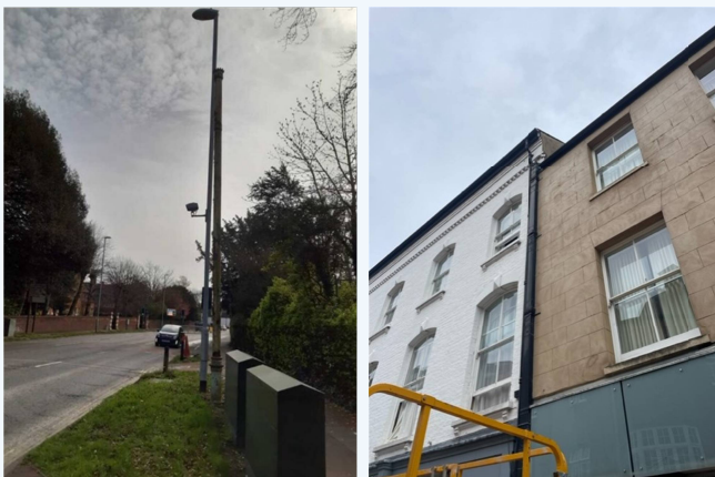
Figures 3.17 & 3.18 Examples of current vents in public rights of way and connected to dwellings/offices.
